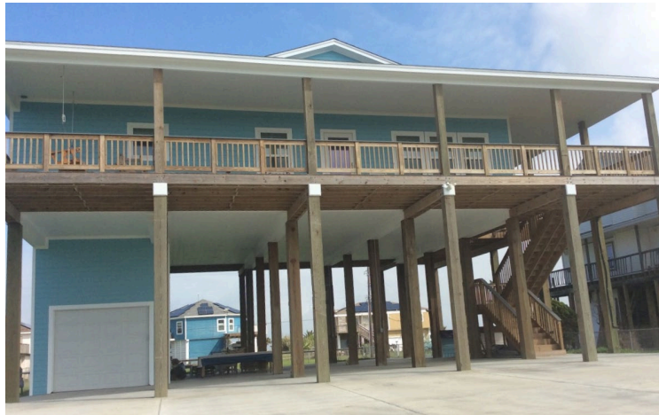
Figure 9. A Building Elevated on Posts/Piles with an Enclosure used for Parking
